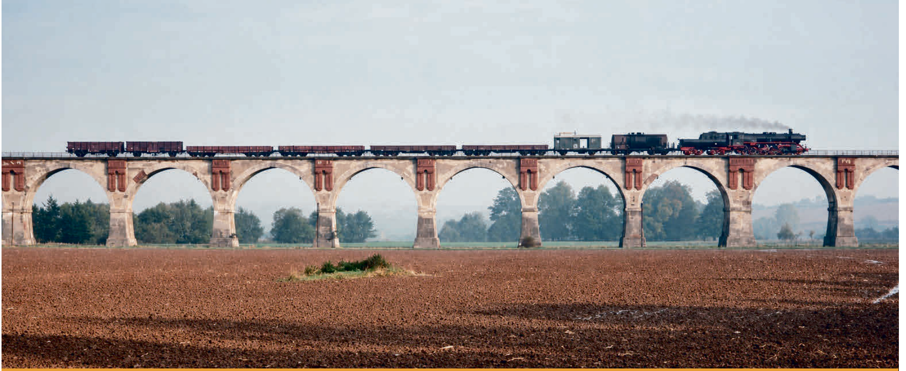
Viadukt in Frohnsdorf.
